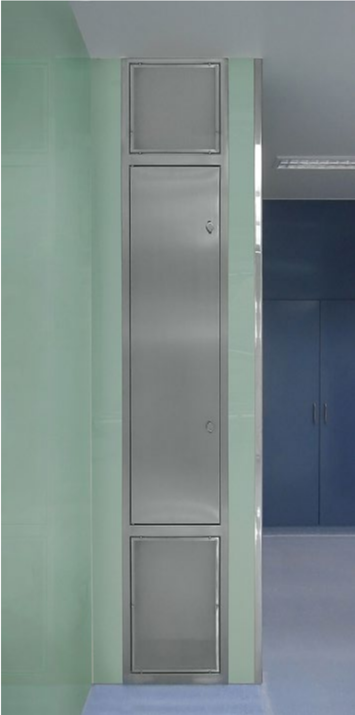
Exhaust air cabinet including fluff separator and inspection door
